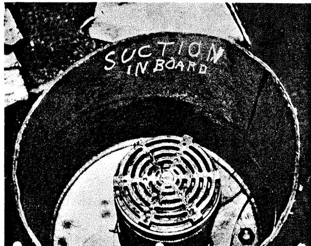
Figure 5. Suction inboard valve.
