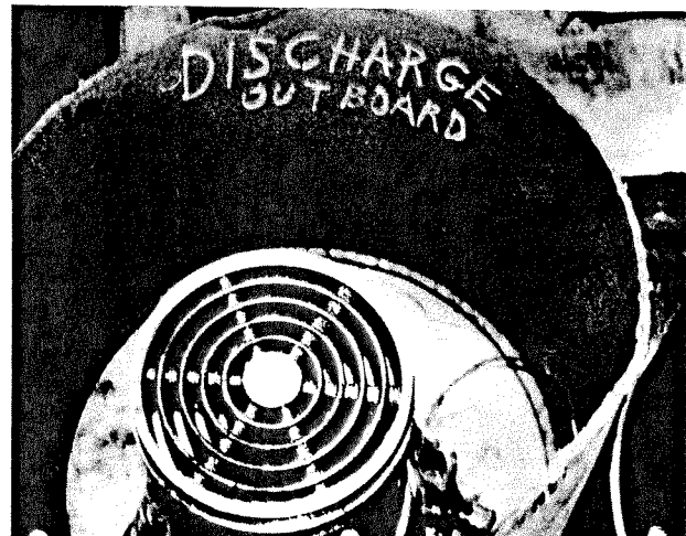
Figure 3. Discharge outboard valve.
